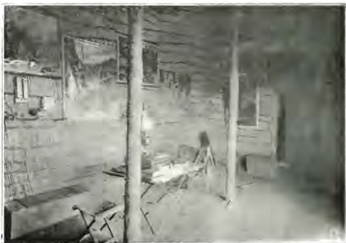
INTERIOR OF MISSIONARIES' HOUSE.
