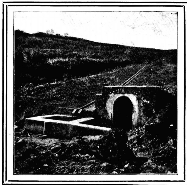
A FOUNTAIN AT THE INDUSTRIAL INSTITUTE, TANGIER.
