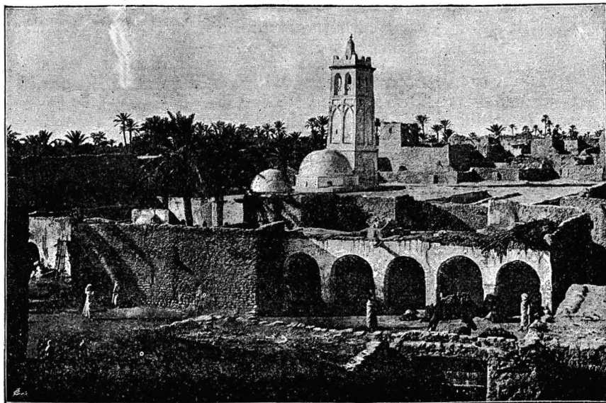
THE MOSQUE OF SIDI OKBA.
