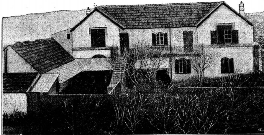
TULLOCH MEMORIAL HOSPITAL, TANGIER, AS SEEN FROM THE ROOF OF HOPE HOUSE (see p. 55).
