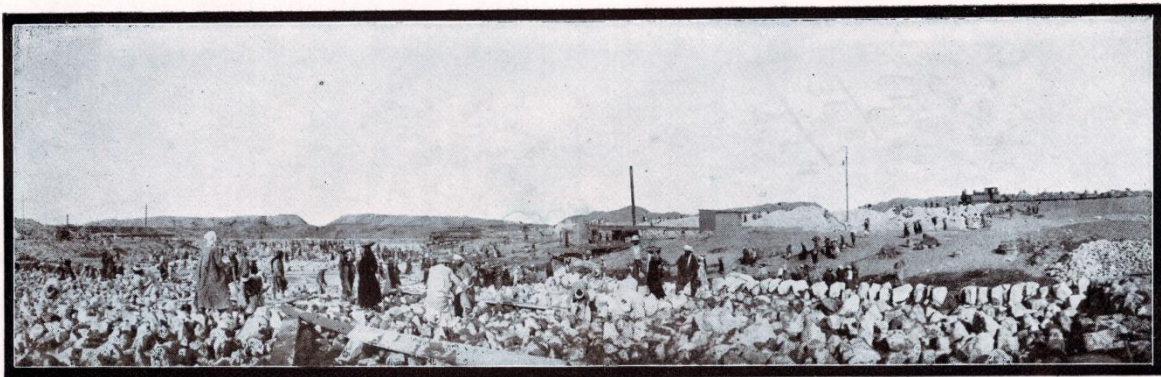
BUILDING THE BARRAGE OVER THE NILE AT ZIFTA.
