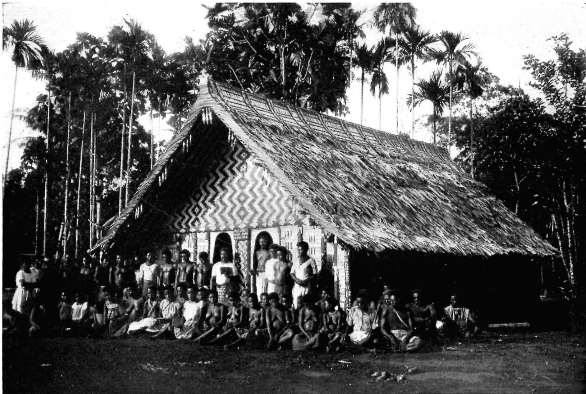
SCHOOL AT BINA, LANGA-LANGA LAGOON.
