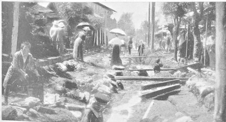
MAIN STREET AFTER THE FLOOD.
