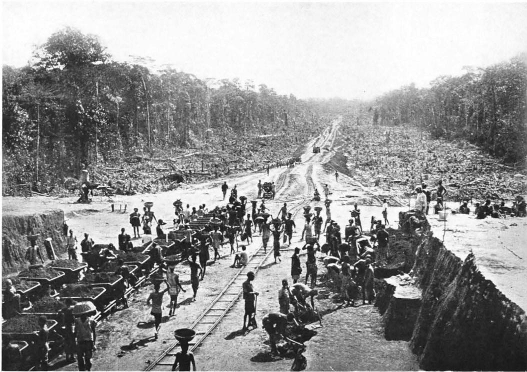
RAILWAY CONSTRUCTION THROUGH THE IMO SWAMP
