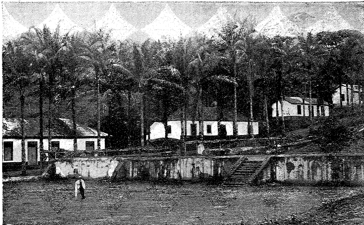
Main Buildings of Angola Plantation
