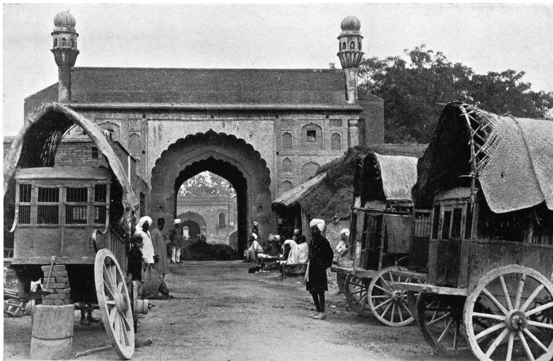
OLD GATEWAY—ENTRANCE TO NEW HOSPITAL AT KARNAL.
