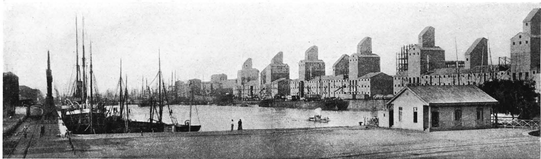
DOCKS AND GRAIN ELEVATORS AT BUENOS AIRES, ARGENTINA
