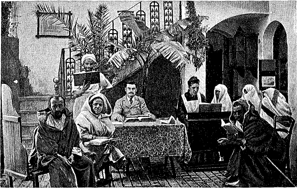
Interior of Tulloch Memorial Hospital.
