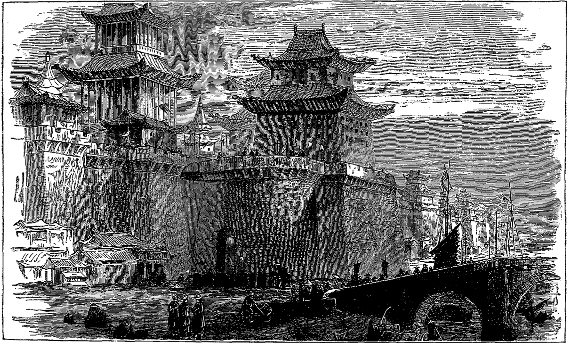
WALL OF PEKING.
