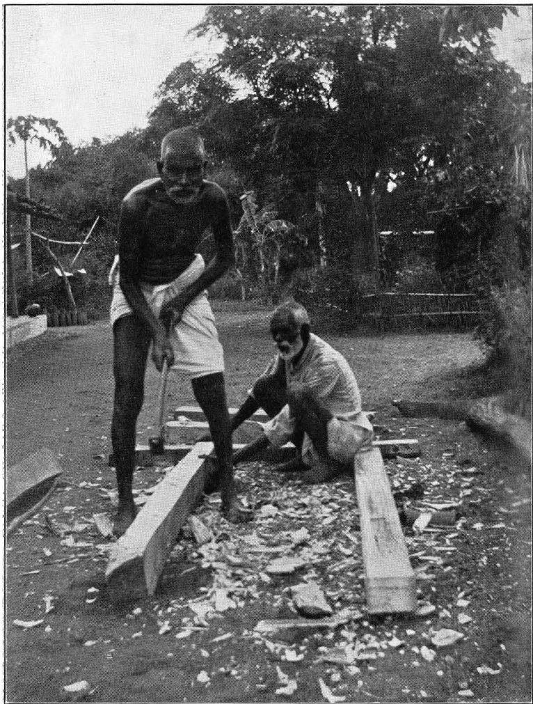
INDIAN CARPENTERS AT WORK
