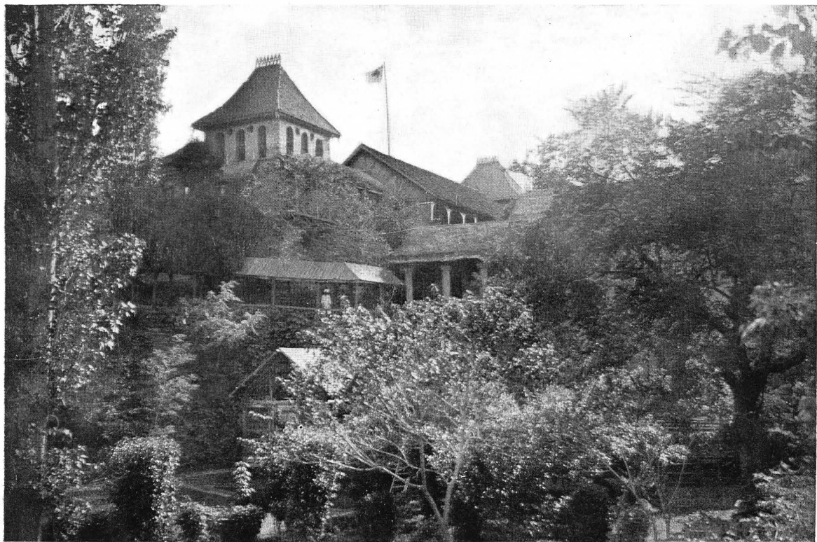
18. CENTRAL TOWER, MISSION HOSPITAL.
