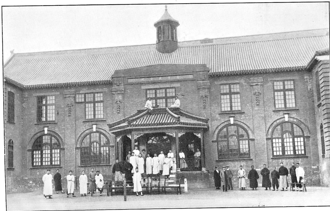
The Men's Hospital, Tai Yuan Fu : North Aspect
