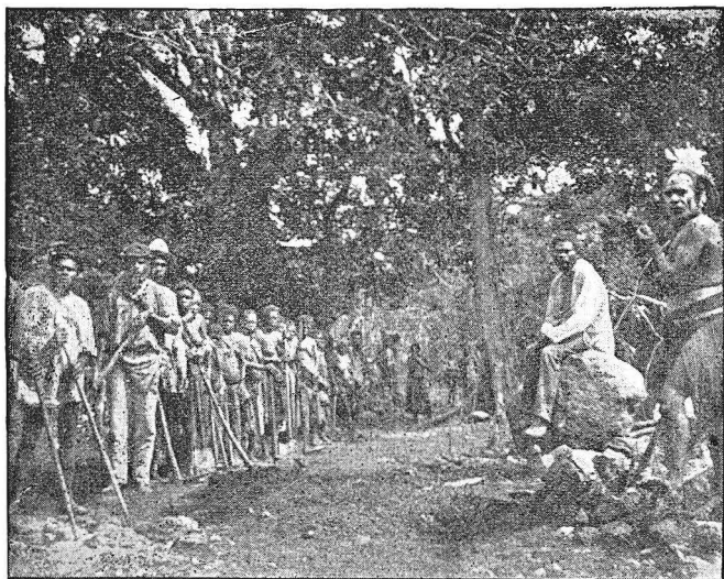
ROAD-MAKING ON TONGOA.
