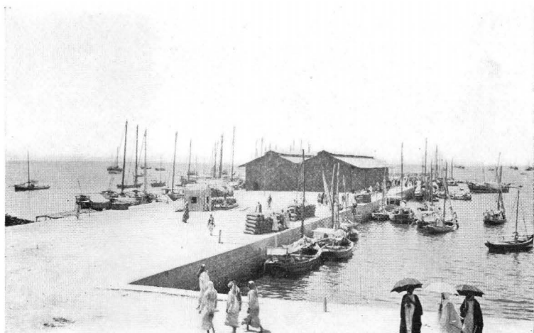
THE NEW PIER, BAHRAIN
