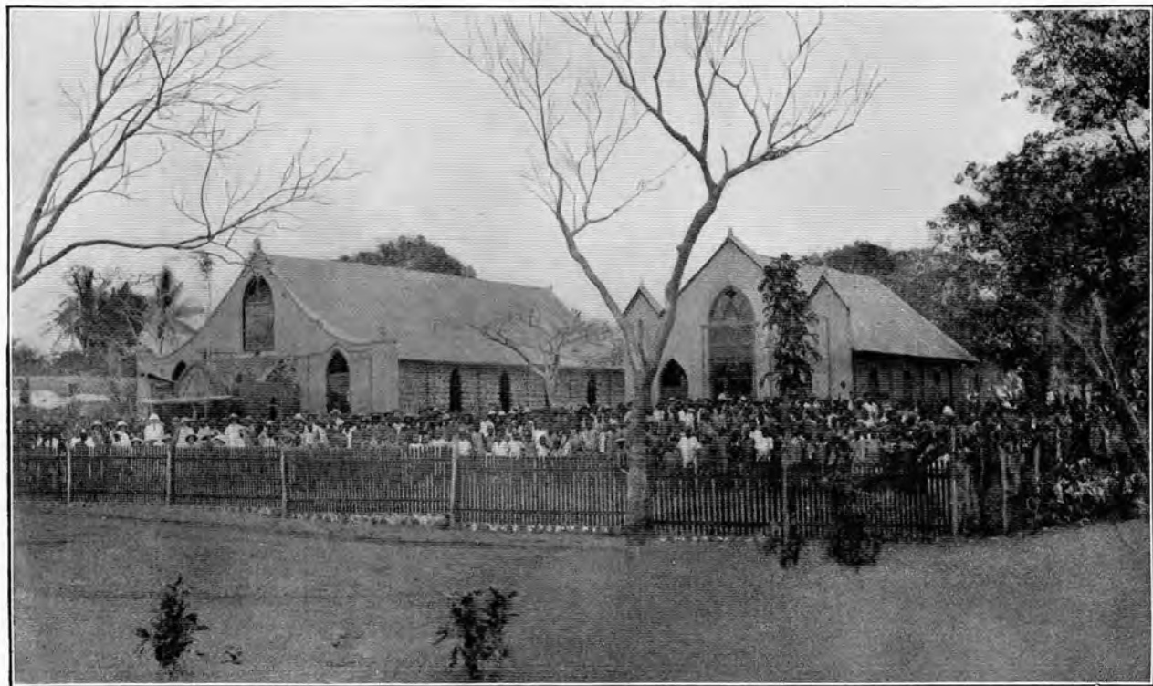
SAN SALVADOR CHURCH ( left ) AND SCHOOL HOUSE.
