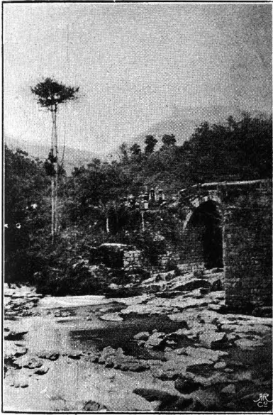
BRIDGE OVER GO-SHI RIVER.
