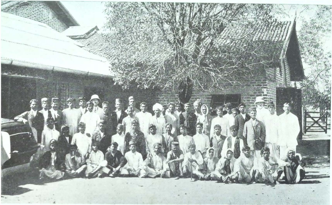
RASULIA INDUSTRIAL WORKS, NEAR HOSHANGABAD, INDIA.
