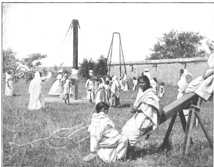
The Playground at Salamatpur
