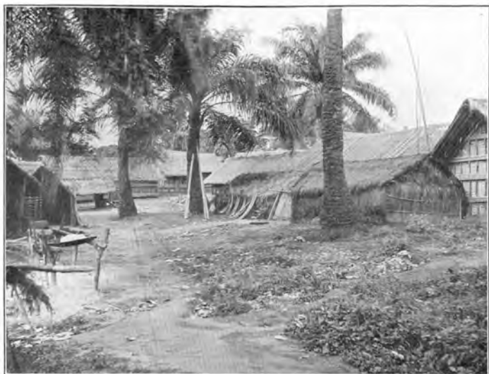
VIEW IN ONE OF THE BOLOBO TOWNS. Photo: G. Grenfell.
