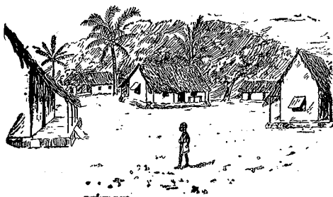
SCHOOL-BUILDINGS AT FRERE TOWN.
