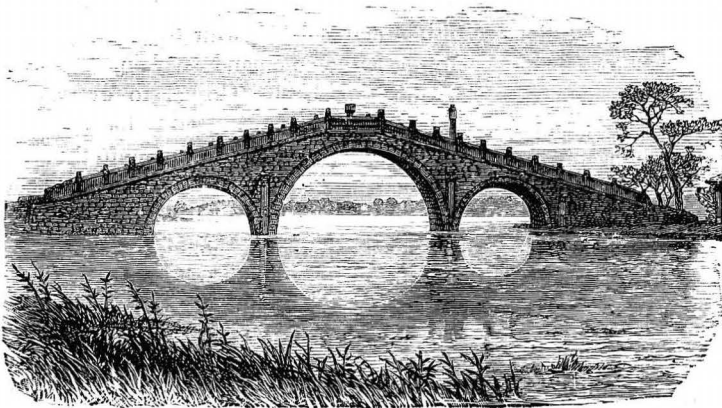
BRIDGE IN CHEH-KIANG.
