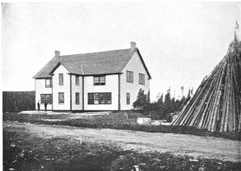
ONE BUILDING OF THE LOCKWOOD SCHOOL AT CARTWRIGHT
