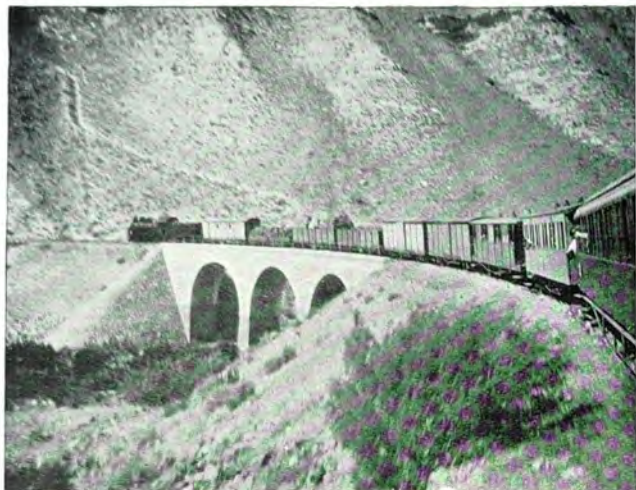
ANCIENT VALLEY OF YERMUK, NEAR WACÛSA MODERN PART OF NEW LINE — HEJÂZ, ARABIA
