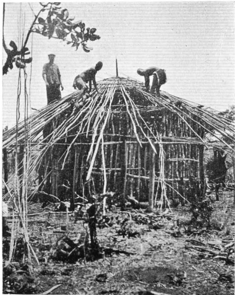
BUILDING A HUT
