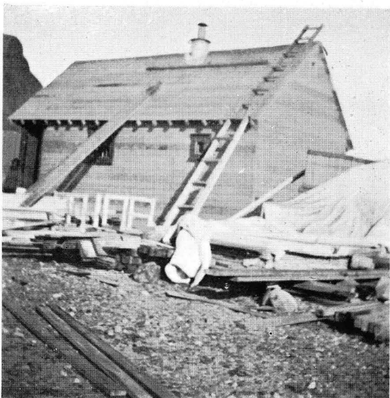
Building the Moffet Inlet mission house
