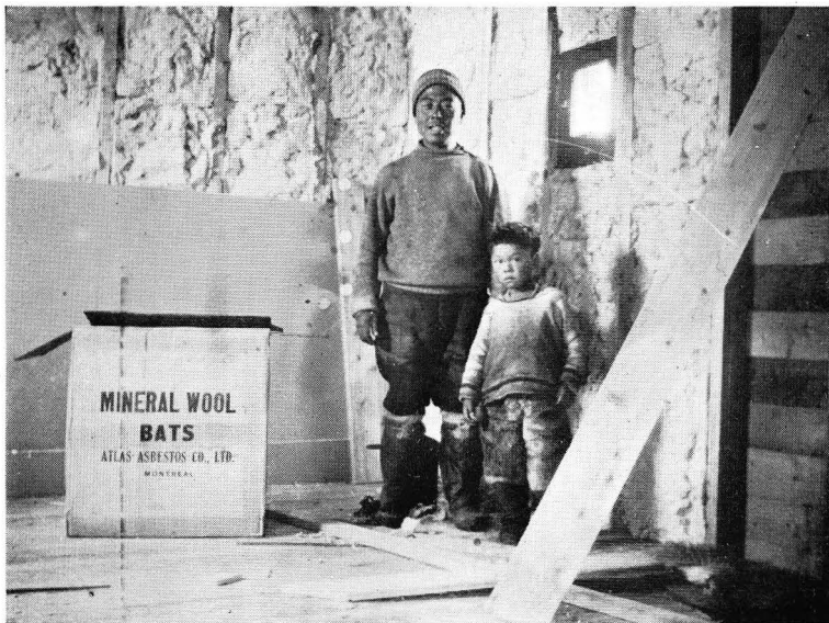
Building the Moffet Inlet mission house
