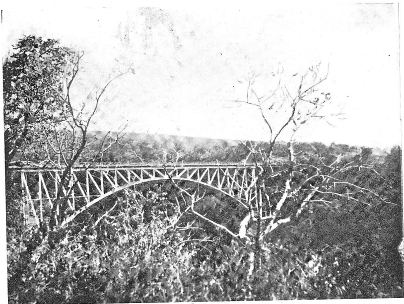
BRIDGE AT VICTORIA FALLS.
