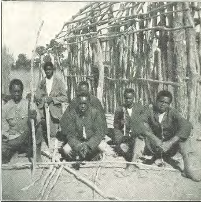
BUILDING A SCHOOL-CHURCH AT AN OUTSTATION.
