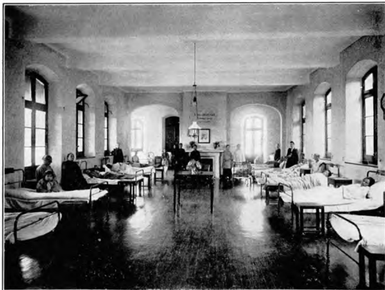
Exterior and Interior Views.
