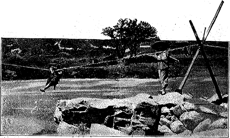
ROPE BRIDGE NEAR TA-TSIEN-LU.
