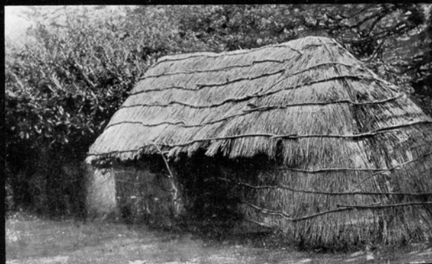
THE THREE STAGES OF MAKING LIVINGSTONE'S LAST HUT IN THE RAIN, THE LAST BEING THE ACTUAL STRUCTURE AS RECONSTRUCTED BY THE VERY MEN WHO MADE THE ORIGINAL ONE.
