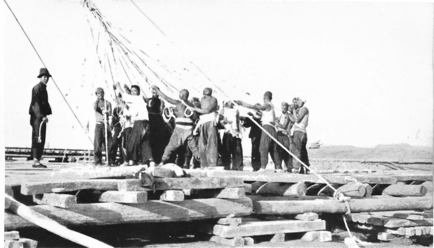
BUILDING TOGETHER— ACCORDING TO PLAN
