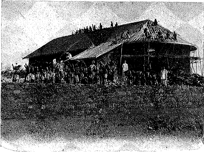
Lusadia Church: Congregation laying the Tiles
