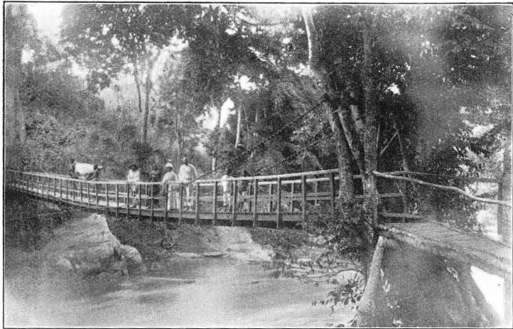
STATE BRIDGE OVER THE LUVU RIVER
