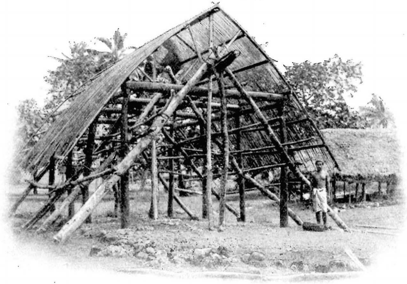
BEGINNING TO BUILD A SAMOAN HOUSE.
