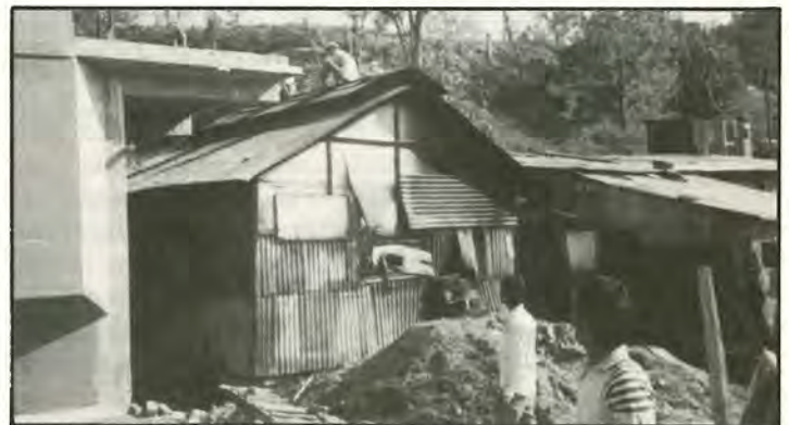
(top left) New hospital buildings (above) Old building before demolition
