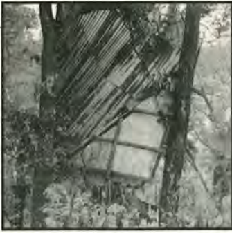
The hostel roof blown onto teak trees
