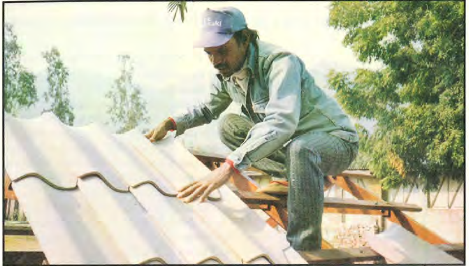
Testing and demonstrating lower cost concrete roofing tiles in Nepal
