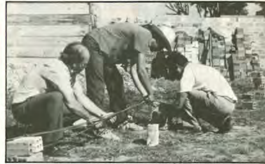
Pastor and church members start building work
