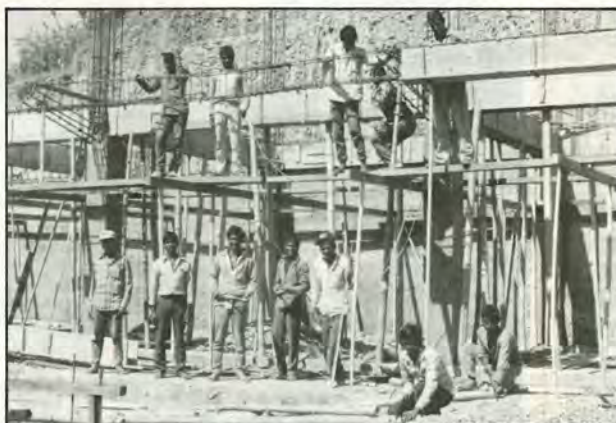
Working on the Mizo Centenary Building
