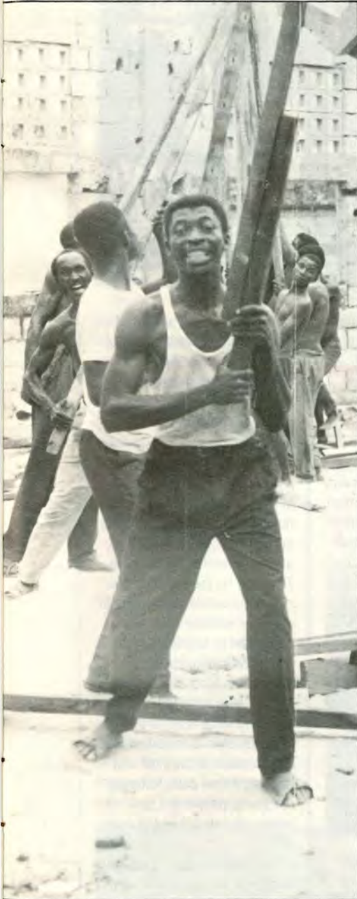
Putting on the roof at Kingabwa
