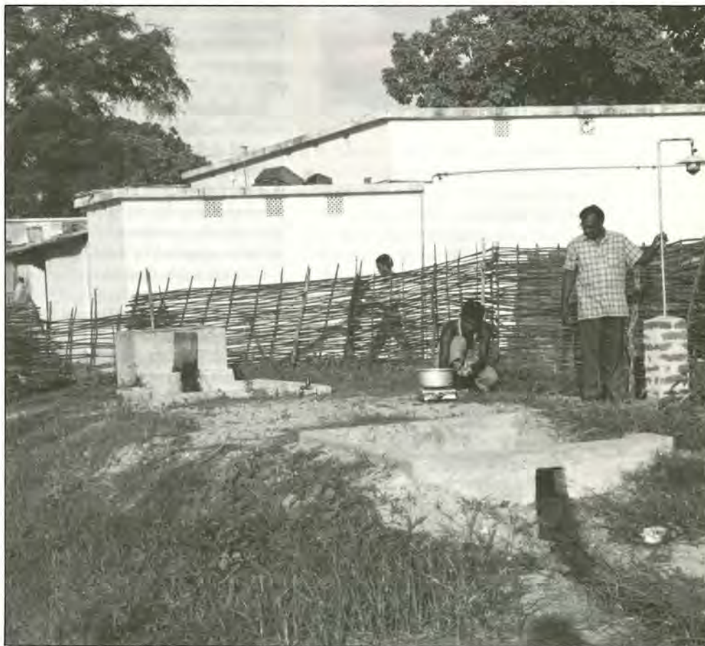
Biogas plant running a stove and light
