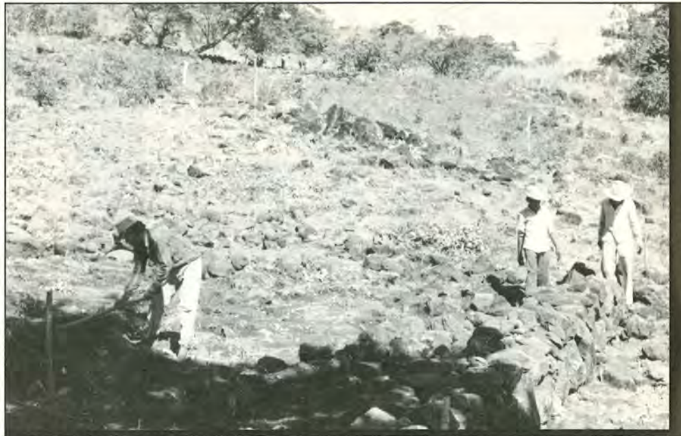
Preparing the ground for resettlement in Agua Caliente
