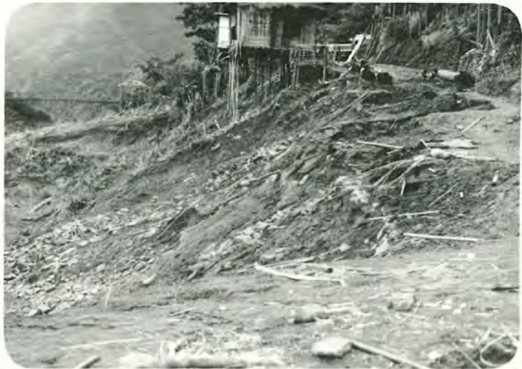
Roads destroyed by flood
