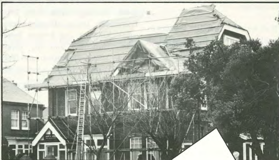
South Lodge, awaiting the builder
