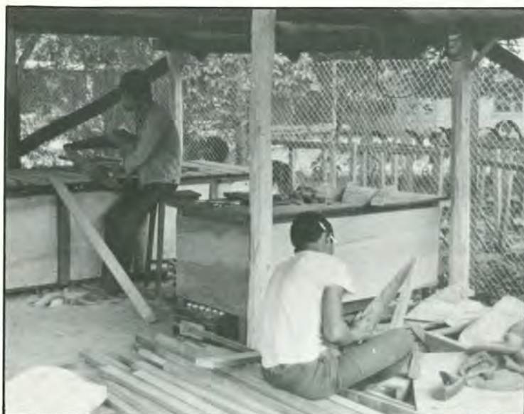
Preparing roof timbers, Butwal
