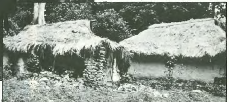
Example of bad thatching, left, good thatching right
