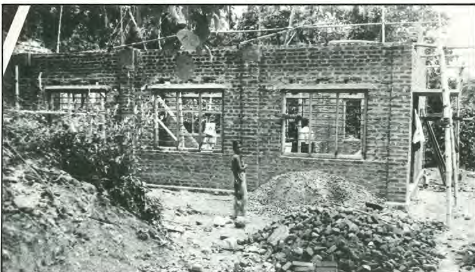
Church being built
