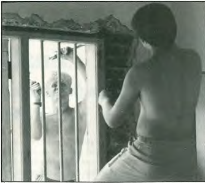
Knocking out a window frame to make way for a doorway
