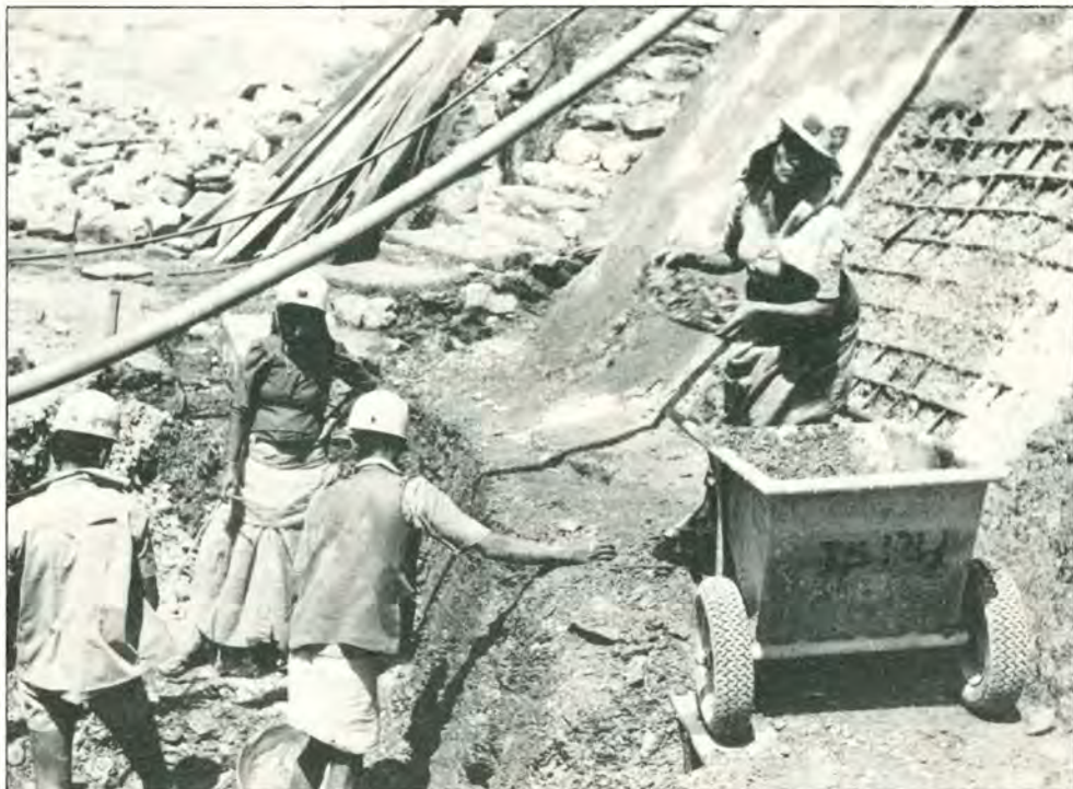
Men and women excavating foundations
