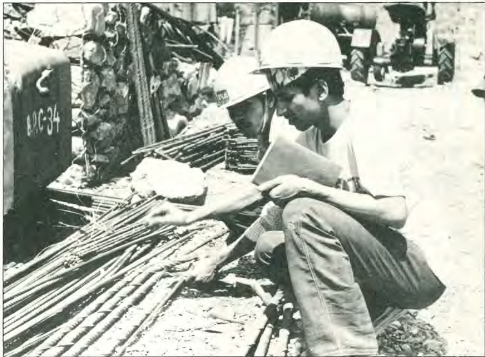
Checking steel rods – some broke while bending
