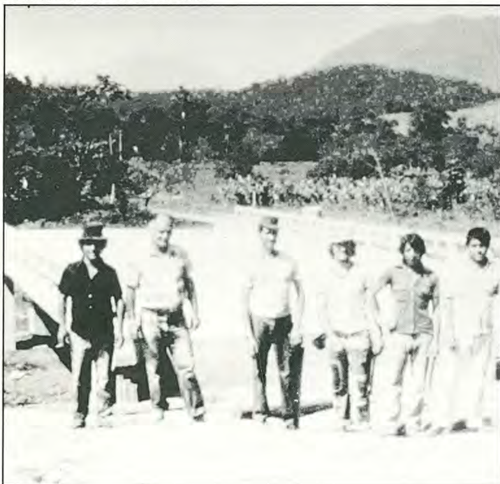
Construction new road in the Litoral
